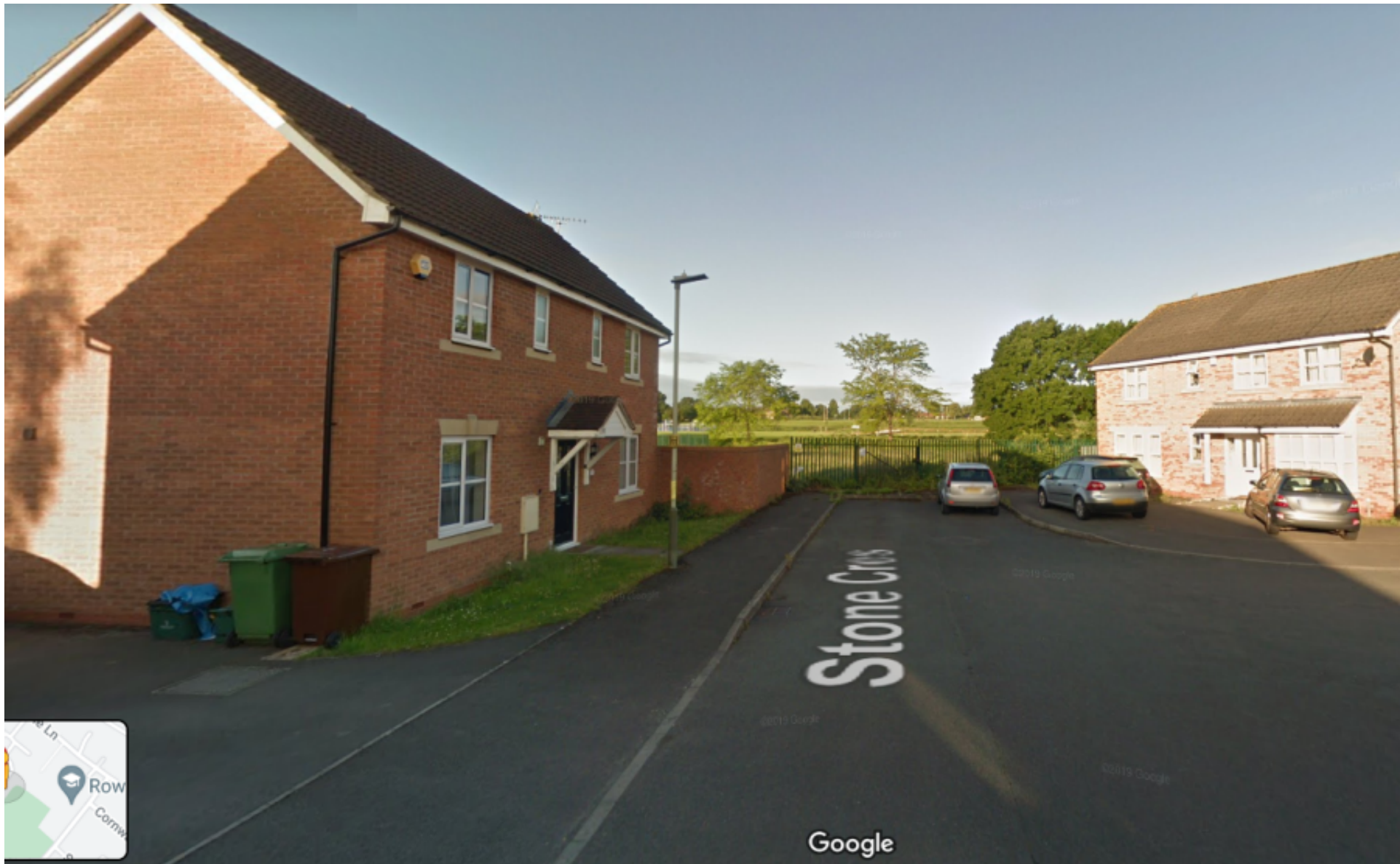
Google maps image of entrance to the application site from Stone Crescent
